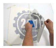
4. Carefully place the cut vinyl graphic against the surface and squeegee firmly in both vertical and horizontal directions, starting from the center and working outward. The squeegee should stay in direct contact with the surface of the vinyl as much as possible in order to prevent air bubbles. SEE FIG. 4.
